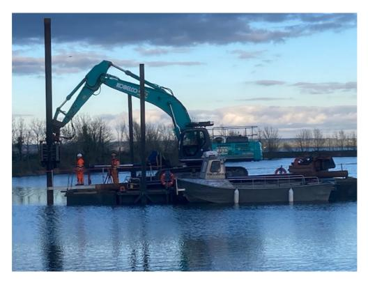
Note that the barge is 15 metres long by 10 metres wide and is moved into position by a dual jet workboat.
